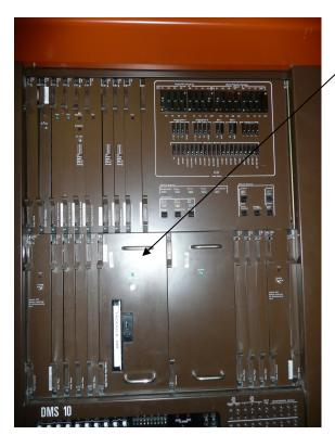
The unit can be used to replace the QIC HP DAT drive in the Nortel DMS10 rack. This is part NTJ1T69A-1.
